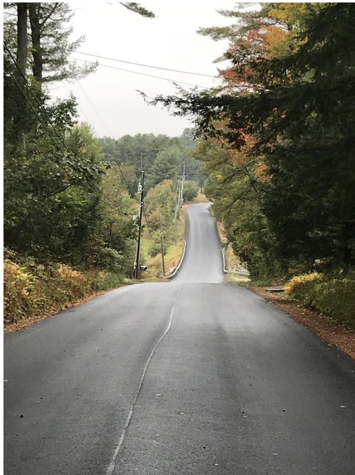
Webster Mills Road after reconstruction in summer of 2019
