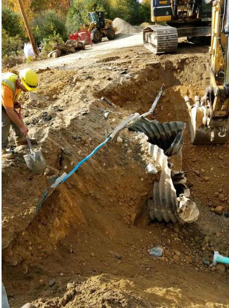
Work on King Road in summer of 2018
